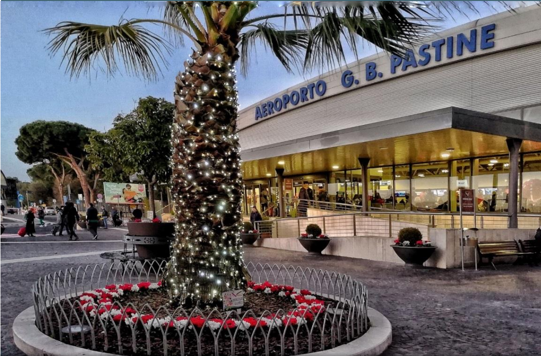
Improvement of the apron in front of the Terminal
